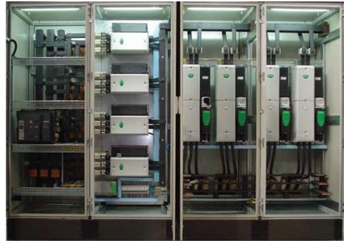
The modular nature of the power circuit allows drive systems to be constructed in non-standard enclosures. For example, it is possible to implement a drive system of between 60 and 2900 hp in an enclosure no taller than 36 in.
